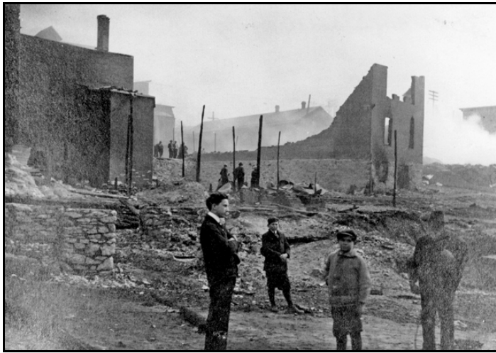
The photo above shows the back of the same buildings on the west side of Main Street looking from Prospect Avenue. The First National Bank is the closest of the two buildings. The Mount Airy Station is in the background.
